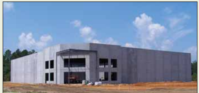
CrossRhodes Shell Building, Bamberg County (photo courtesy of SouthernCarolina Alliance) (Building Inquiry? – Call Kell Anderson, SouthernCarolina Alliance at 803-541-0023)
